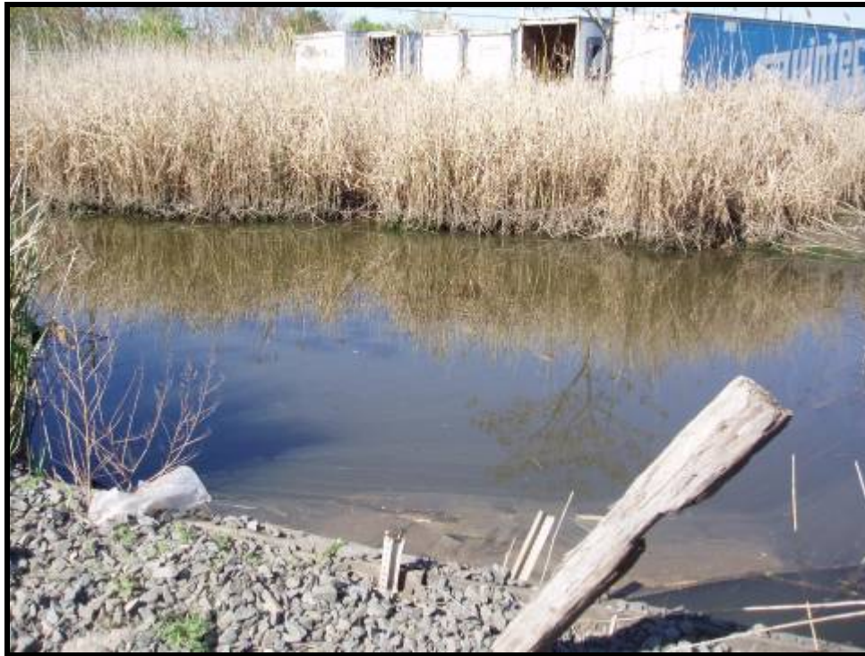
3. Entrance channel to collapsed twin culverts (5/17/05)
