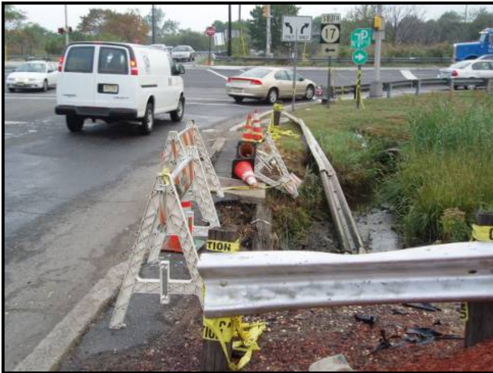
2. Collapsed catch basin located near the intersection of Polito and Rutherford Avenue (10/06/05)
