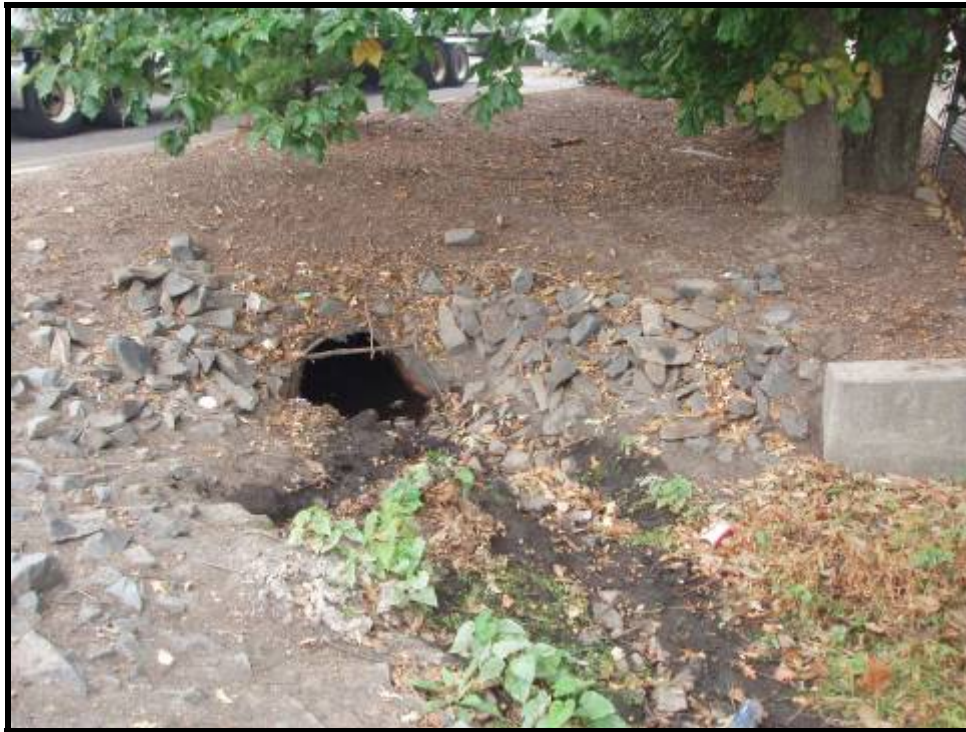
3. Detention basin located at 1 Carol Place (10/06/05)
