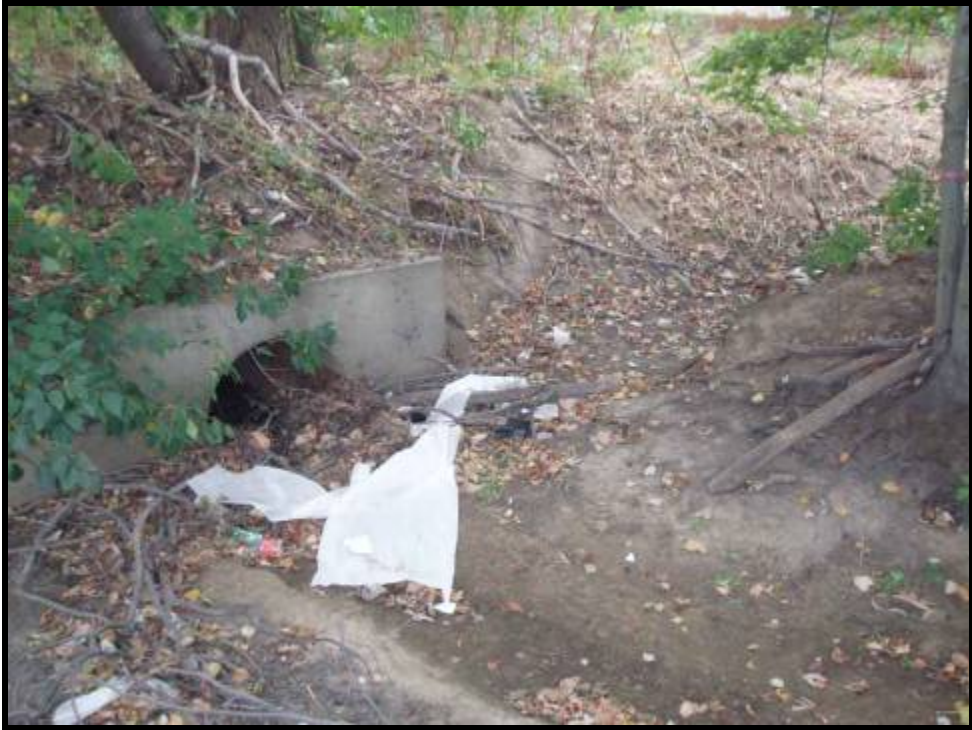
2. Drainage ditch at end of Carol Place (10/06/05)
