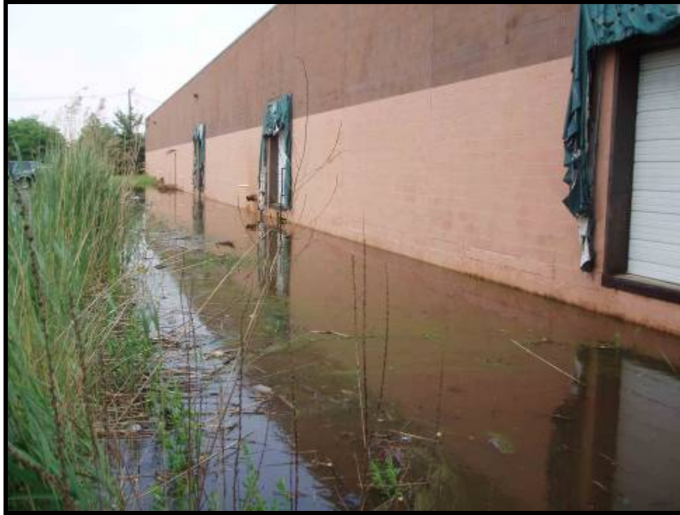
1. Flooding condition behind 360 Murray Hill Parkway (6/10/05)
