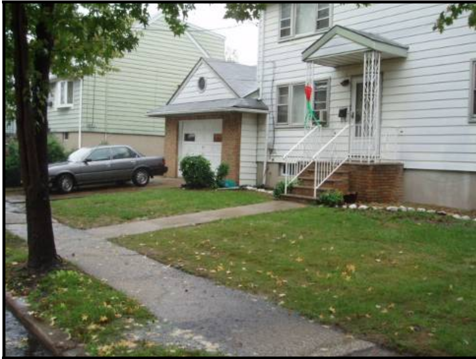
1. Looking at the south side of the property at 176 Louis Street (10/14/05)
