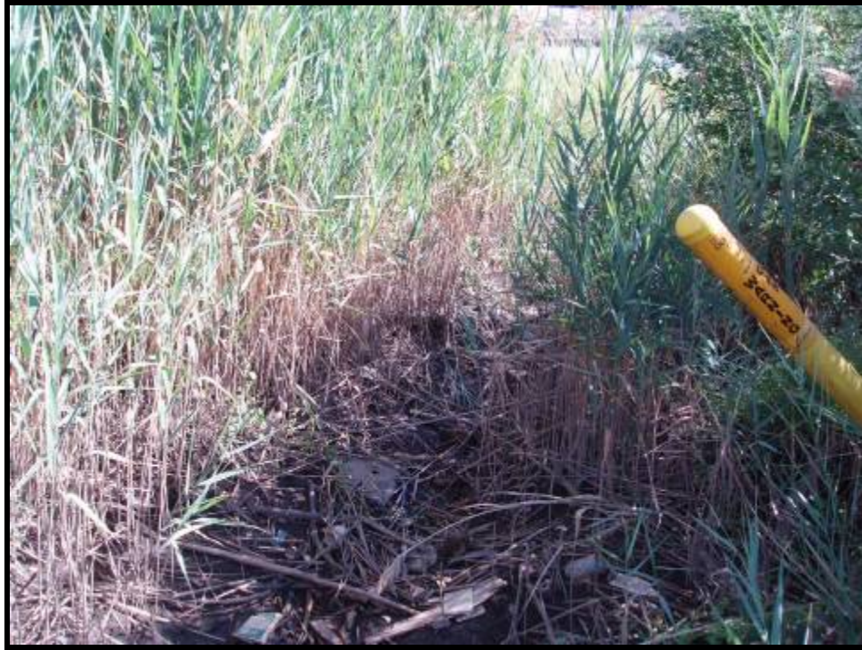
7. View of discharge channel to Hackensack River from above system (Photo 6) (10/06/05) (Note: Gas line warning marker at right)
