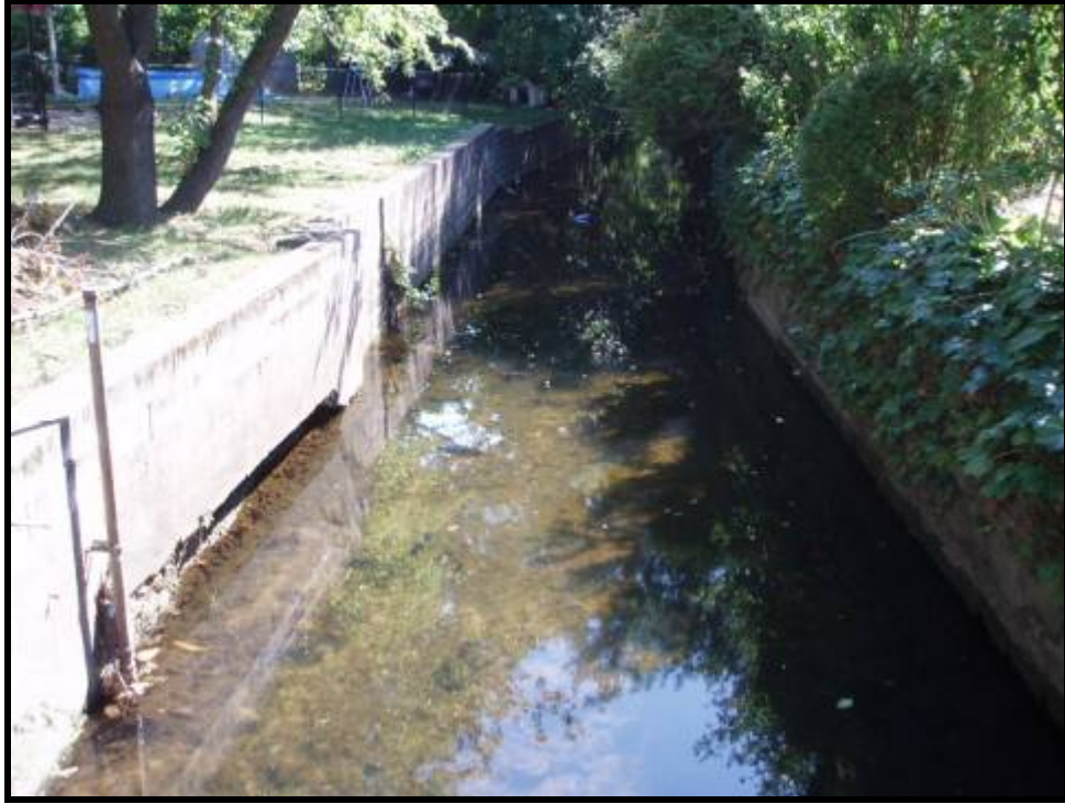
3. Wolf Creek looking Southwest from Clark Avenue Overpass (9/09/05)
