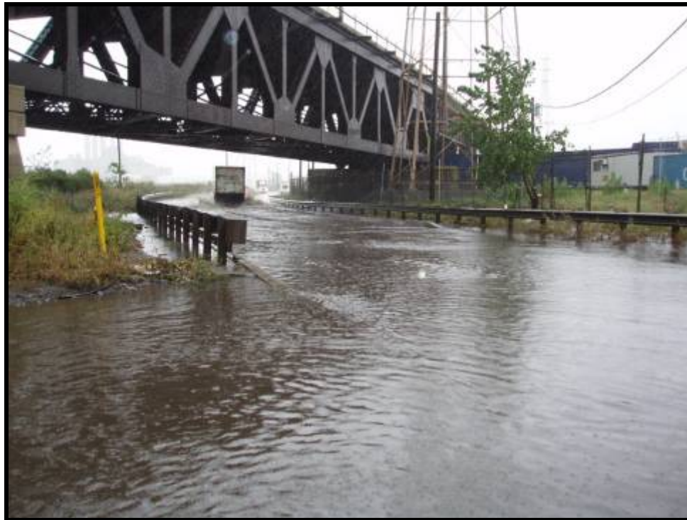
2. Looking Southwest along Fish House Road near CSX rail bridge (10/14/05)
