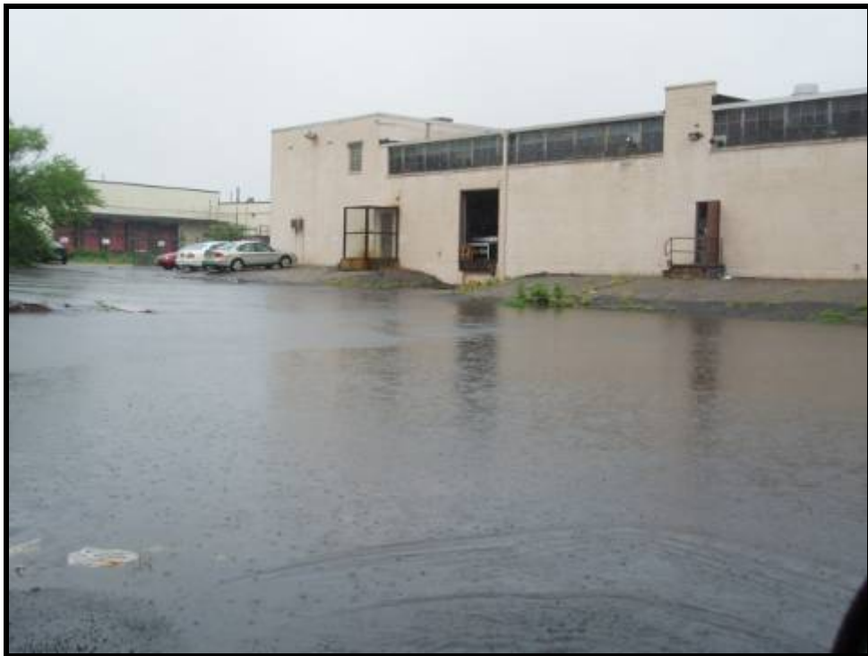
6. Flooding condition behind 705 Commercial Avenue (7/08/05)
