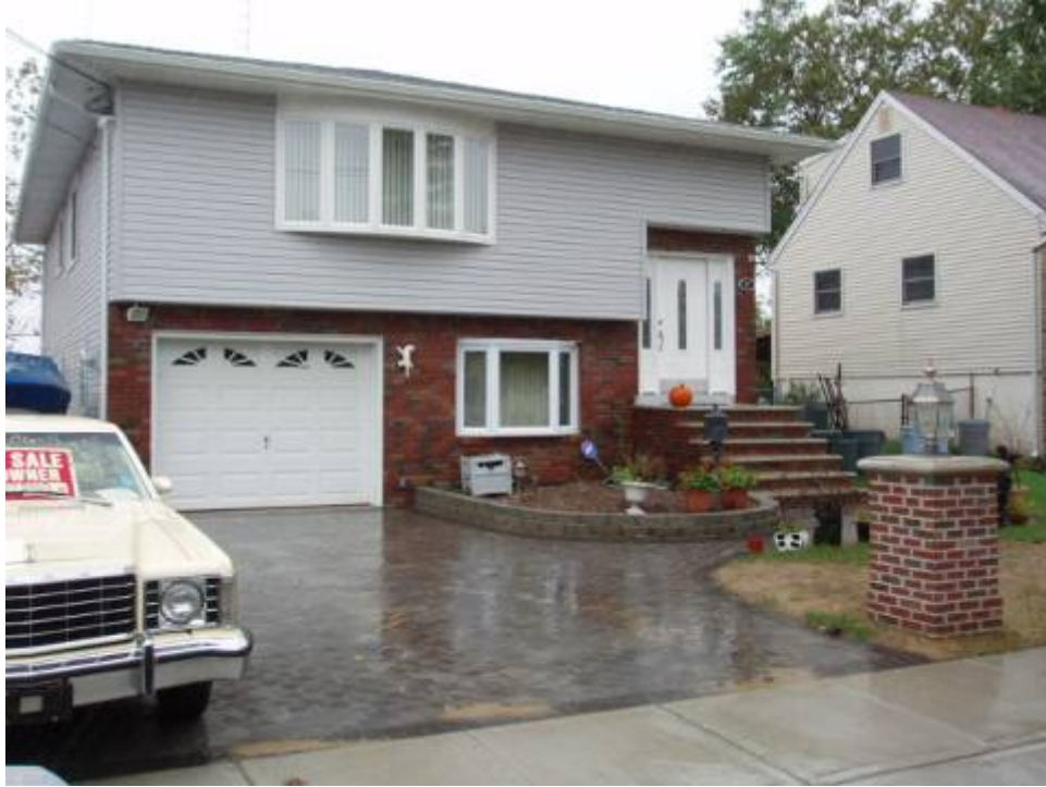
1. Looking at the north side of the property at 67 Huber Street (10/14/05)
