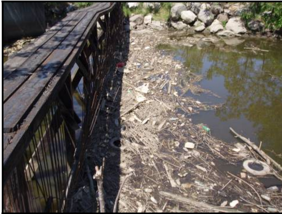
3. Trash rack for East Riser Tide Gate (5/17/05)
