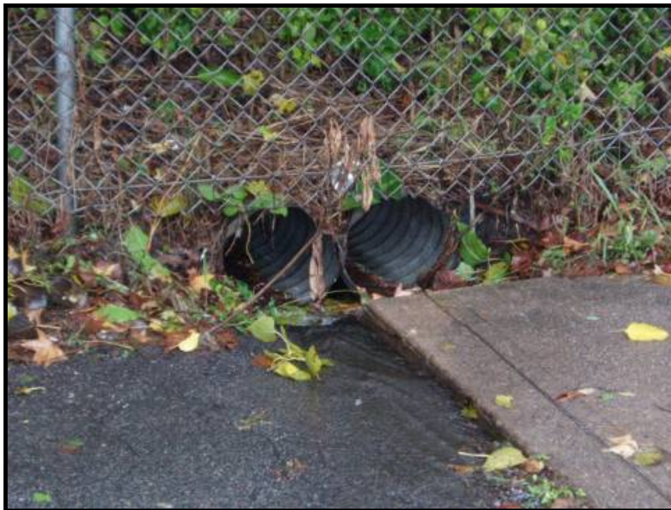
4. Hartwick Street pipe outlet flowing to drainage ditch towards DePeyster Pump Station (10/14/05)
