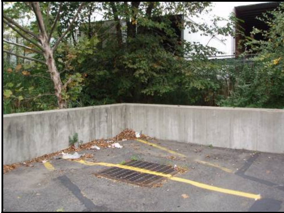
1. Inlet and floodwall at 430 Gotham Parkway (10/06/05)
