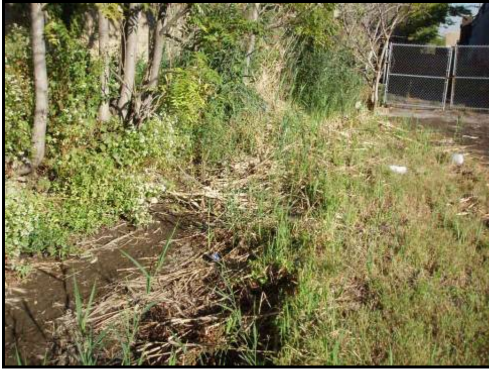
1. Looking downstream at drainage ditch behind 450 Barell Avenue (10/06/05)
