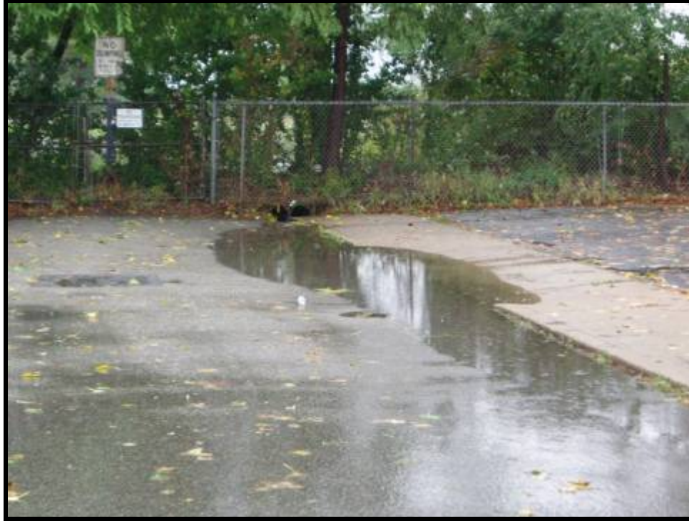
5. Ponding in front of the property at 37 Hartwick Street (10/14/05)
