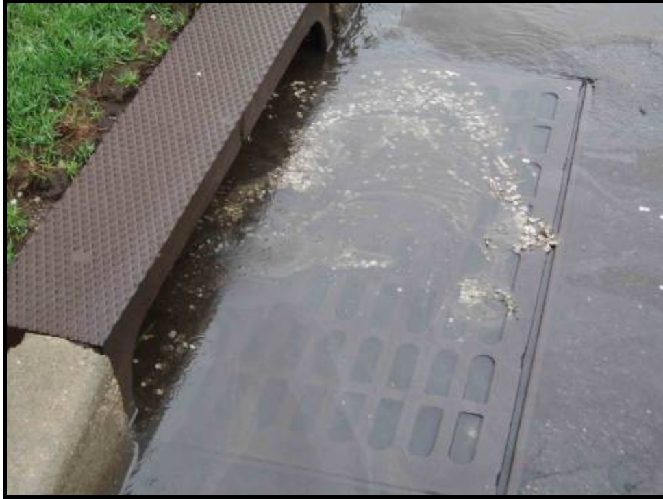
3. Catch basin on 16 th Street at the intersection of Paterson Plank Road and 16 th Street (4/29/05)
