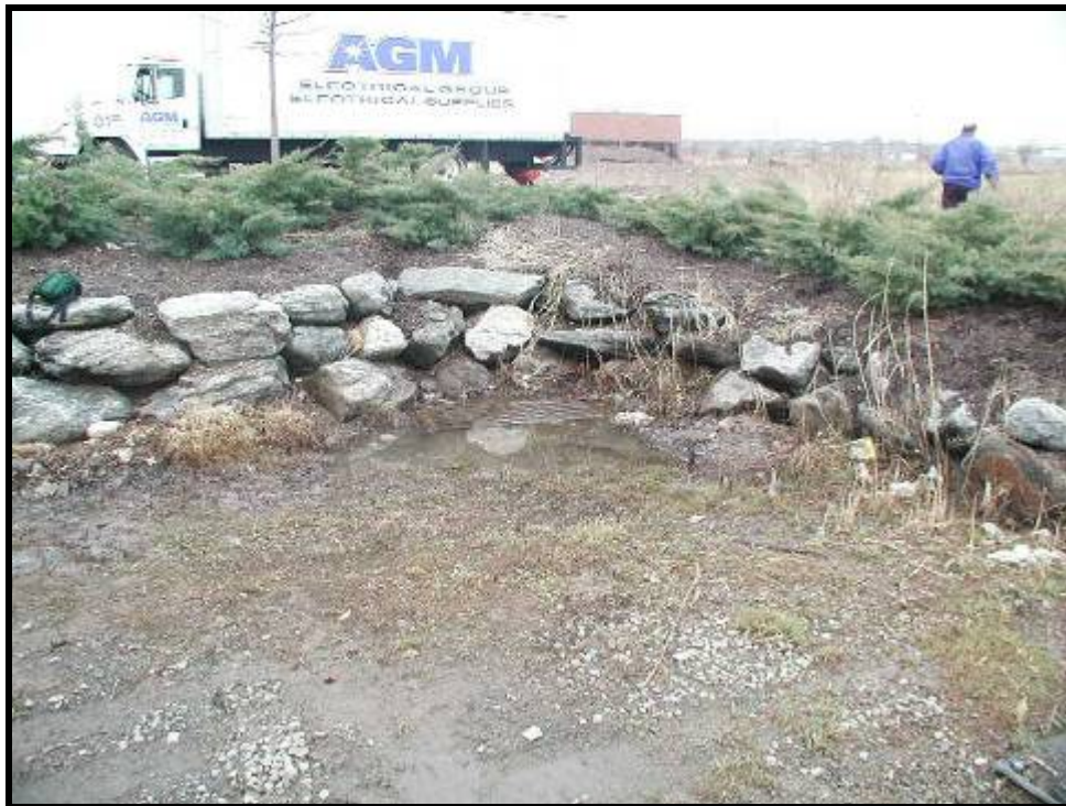
2. Inlet on 758 Paterson Plank Road discharging to above outlet (Photo 1) (3/21/05)
