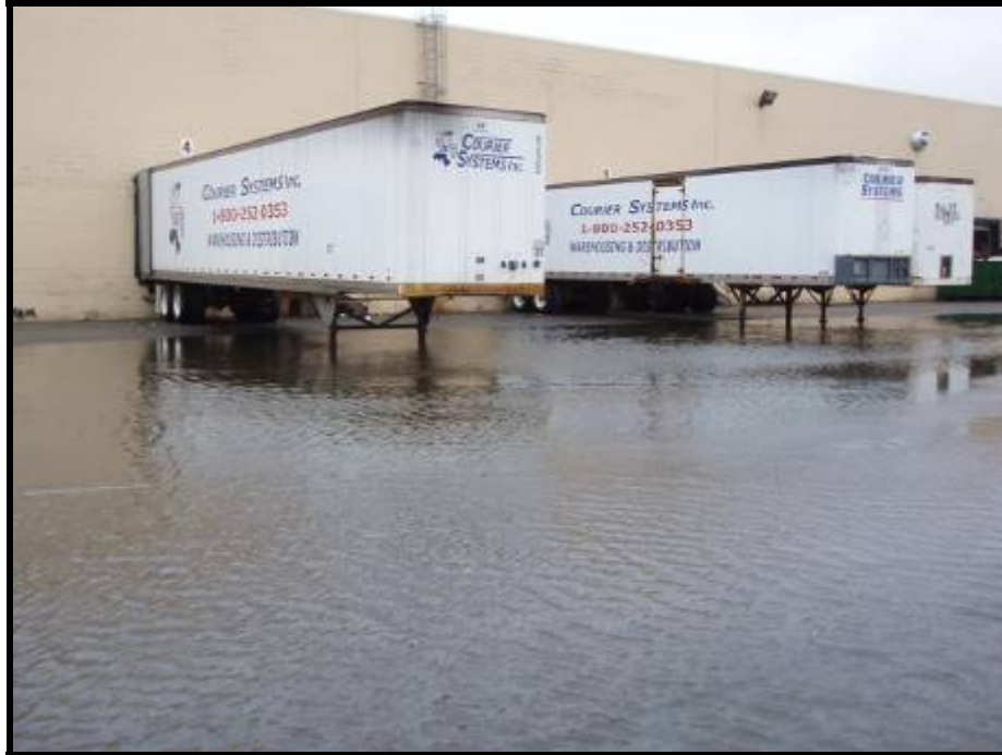
3. Looking southwest towards loading docks (10/14/05)
