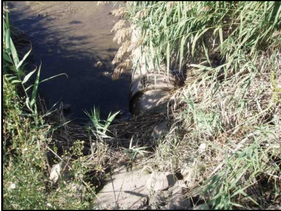
5. Looking at Meadowlands Parkway outfall near Route 3-East entrance ramp (10/03/05)
