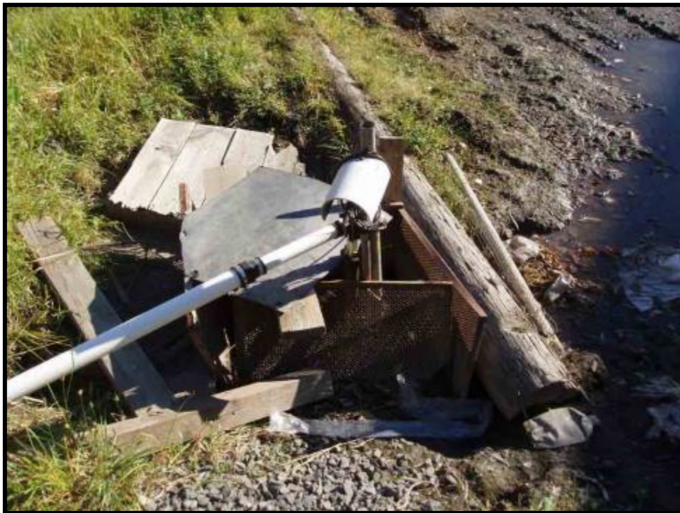
2. Make-shift pump system behind 462 Barell Avenue (10/06/05)
