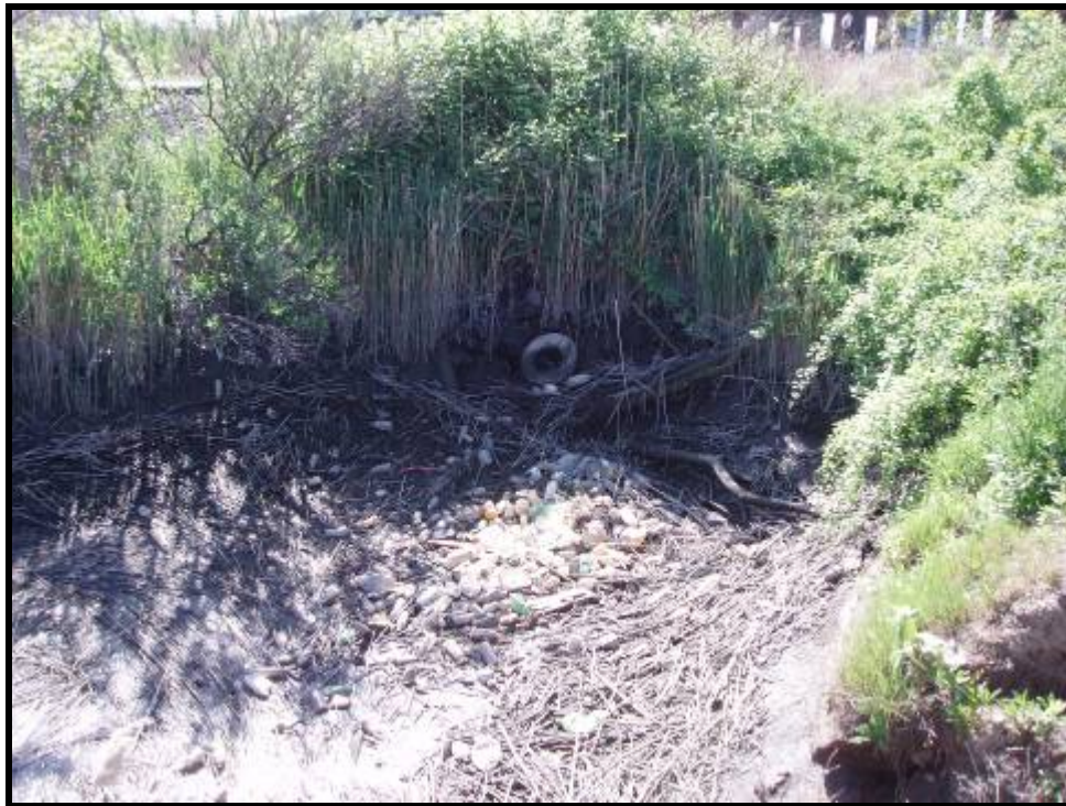
2. Upstream inlets (submerged) to the Rutherford Tide Gates (5/17/05)
