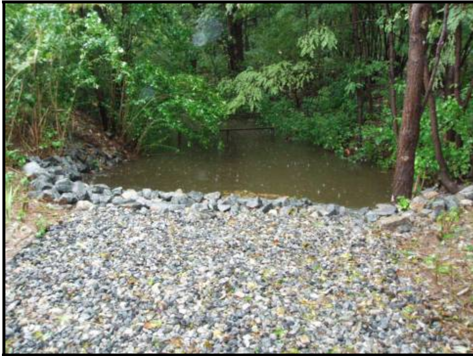
1. Looking upstream of the intake to the DePeyster Pump Station (10/11/05)
