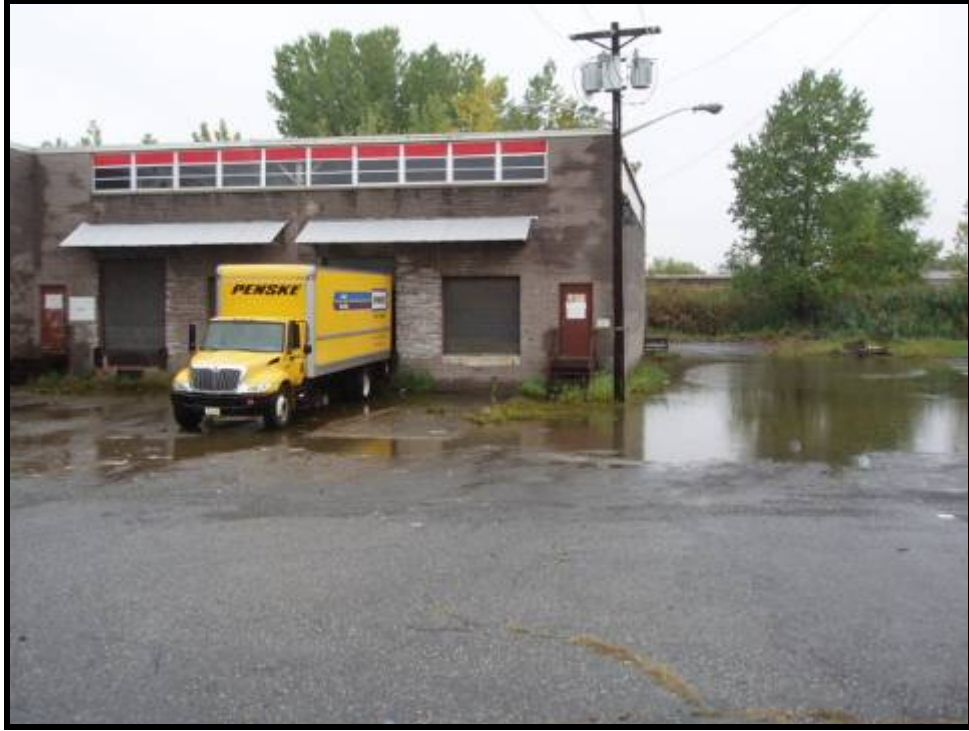
5. Flooding condition at 462 Barell Avenue (10/14/05)
