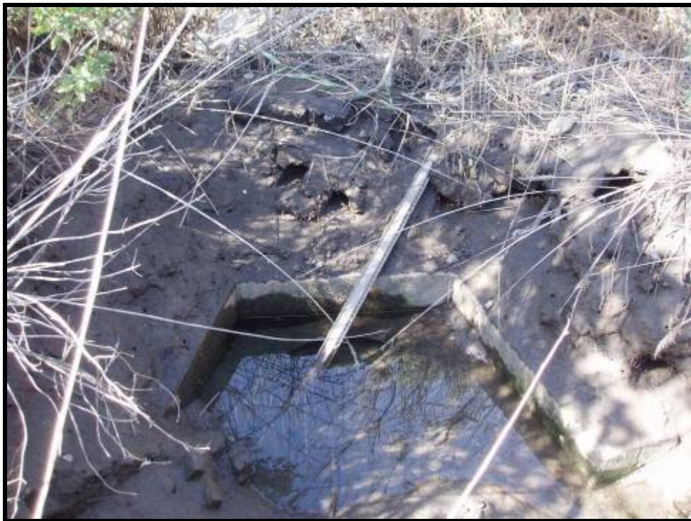
4. Outlet located alongside Fish House Road near the PATH bridge (10/06/05)
