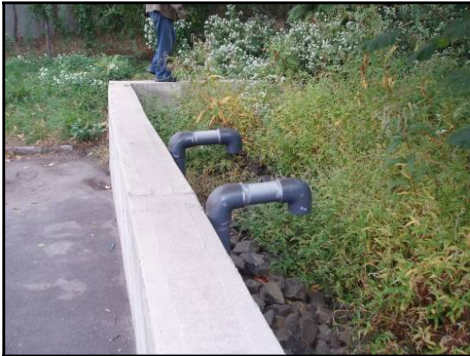
3. Outfall pipes from pump station at 480 Gotham Parkway (10/06/05)
