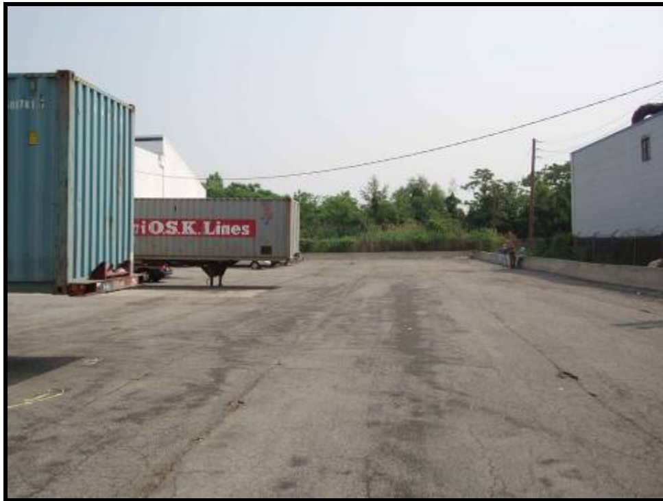
3. Looking Northeast of parking lot towards the floodwalls (6/15/05)
