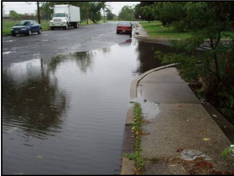
4. Looking West at the clogged inlet on the Michelle Avenue culvert (downstream on left) (10/12/05)
