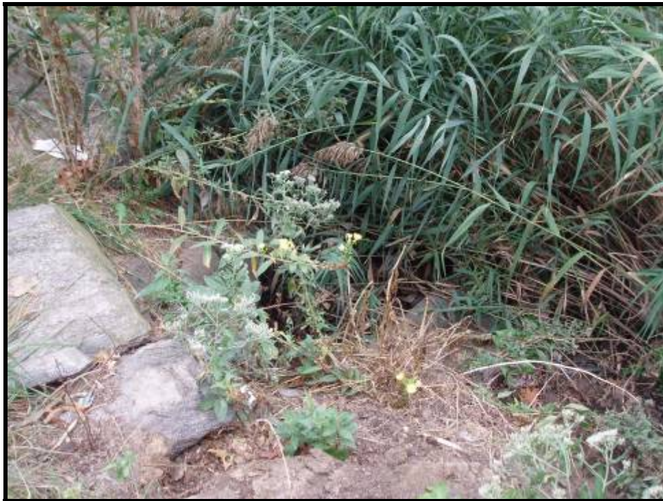
6. Elliptical culvert clogged with debris and vegetation at the rear of 545 Dell Road (10/06/05)
