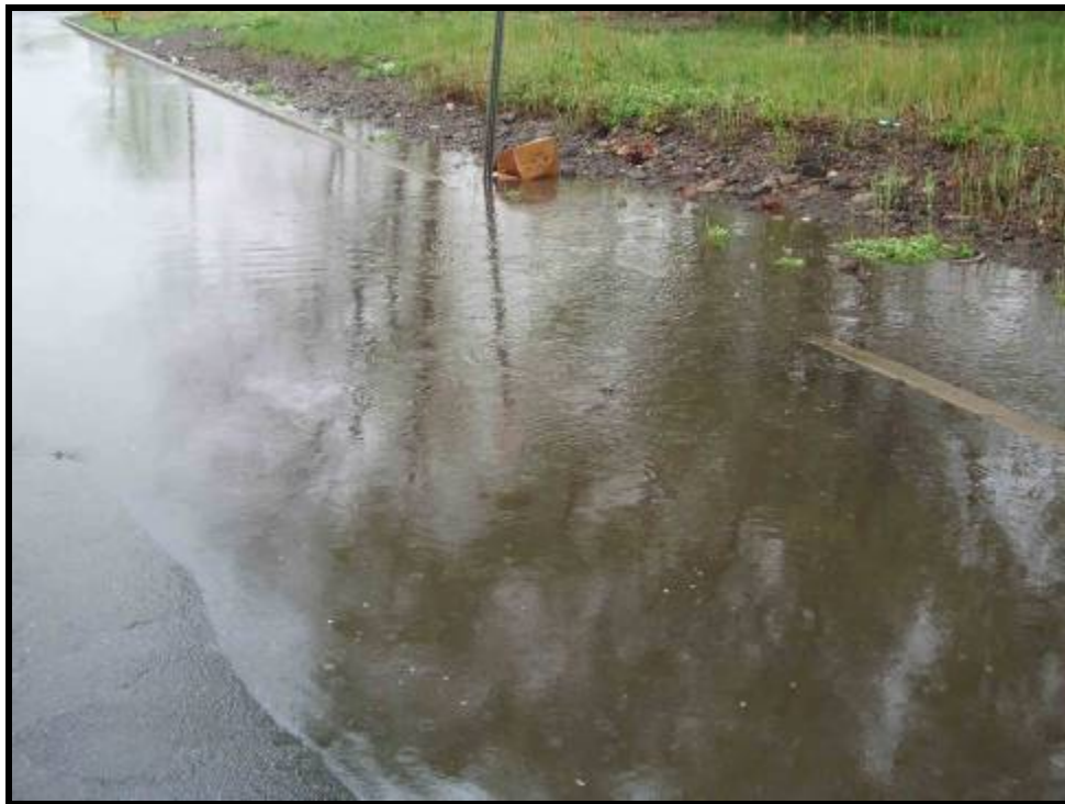
2. Looking Northeast on 16 th Street along side Block 116, Lot 1 (4/25/05)
