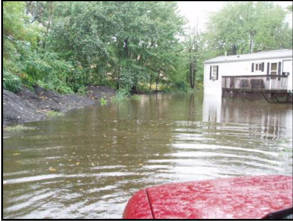
3. Flooding condition along the edge of the mobile home area (10/14/05)
