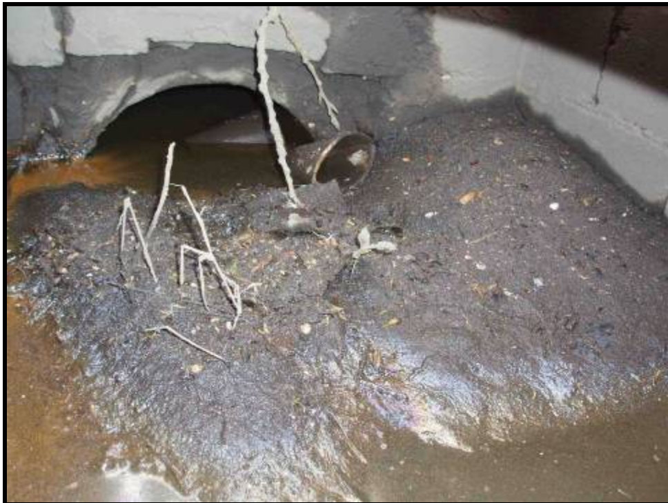
4. Interior of Photo No. 3 catch basin (4/29/05)
