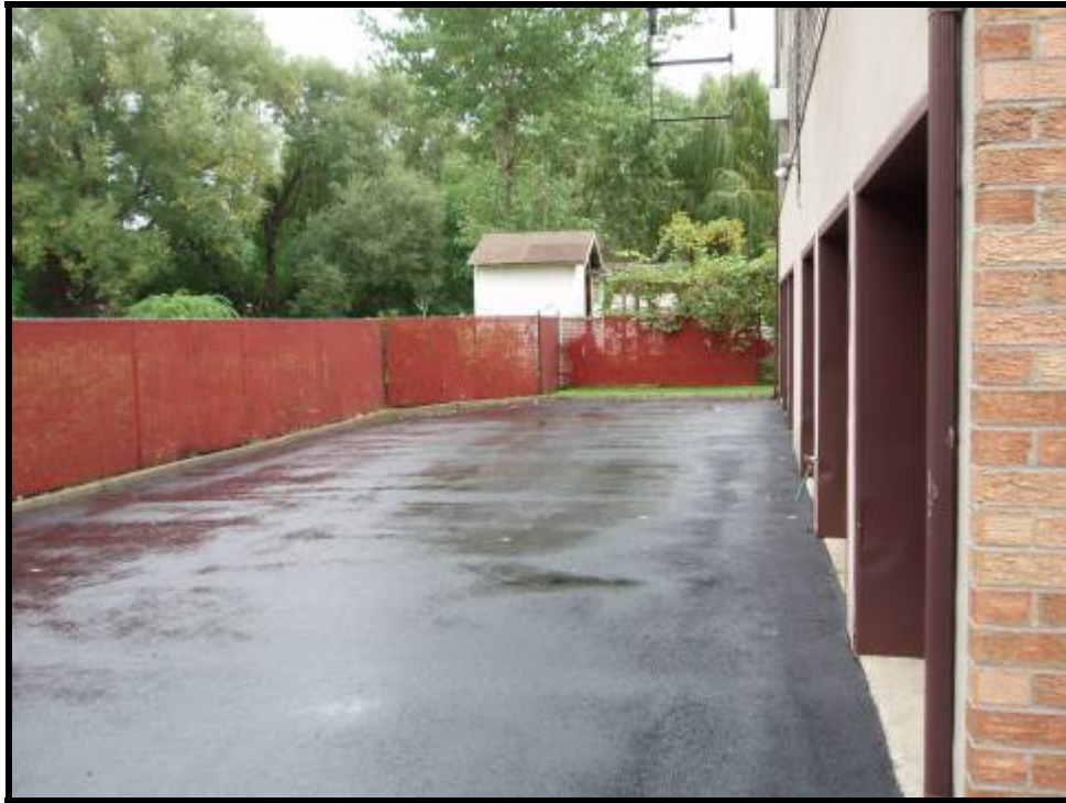
1. Parking area for the residence of 1138B Farm Road where flooding occurs (10/11/05)
