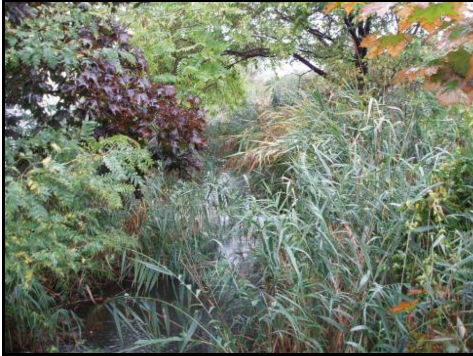
5. Looking upstream at the Michelle Avenue culvert (10/06/05)
