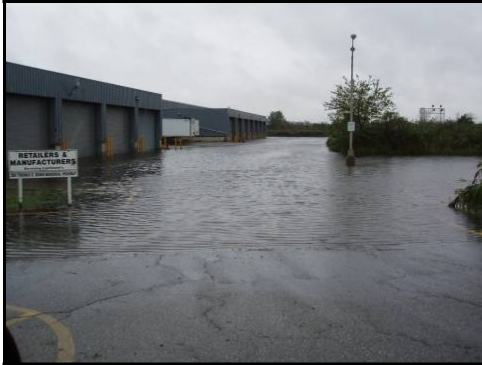
5. Flooding condition in loading docks at 299 Thomas E. Dunn Memorial Highway (10/14/05)
