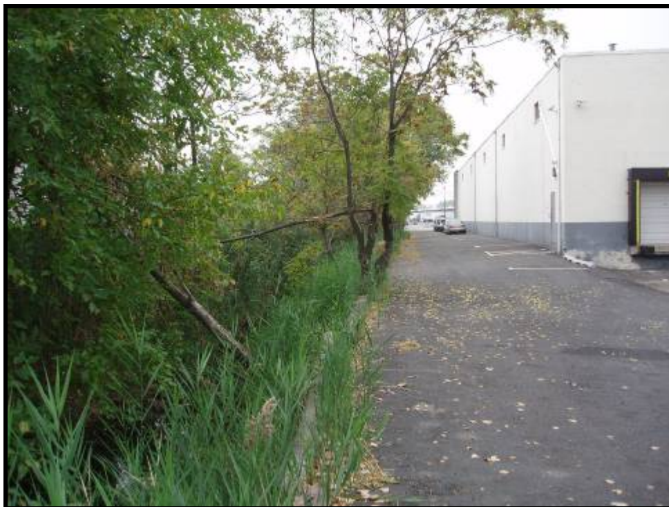
4. Looking downstream at rear of 725 Dell Road (ditch at far left) (10/06/05)
