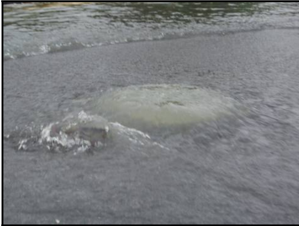
3. Surcharge condition for an inlet on 91 st Street (10/14/05)
