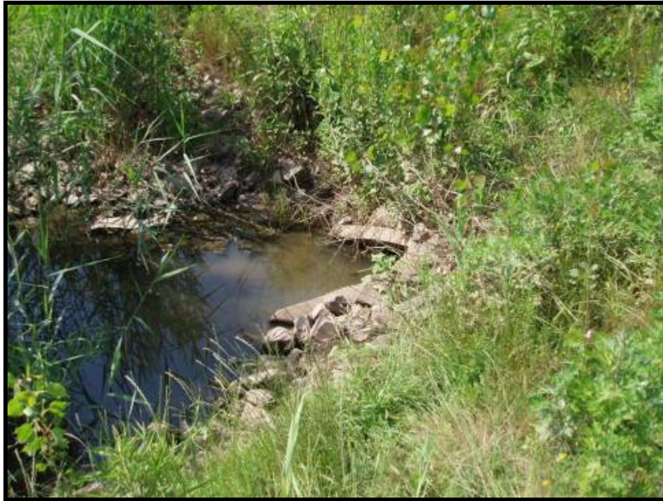
1. Looking at outfall that is connected to the inlet at 758 Paterson Plank Road (6/22/05)
