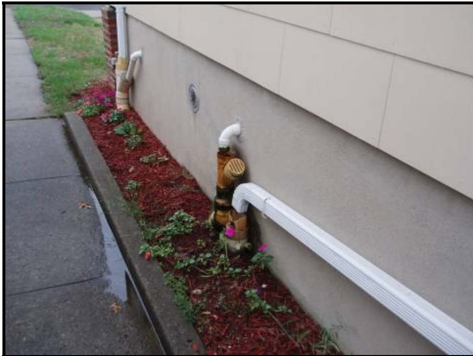
2. Side view of the property at 15 Mill Ridge Road (10/14/05)
