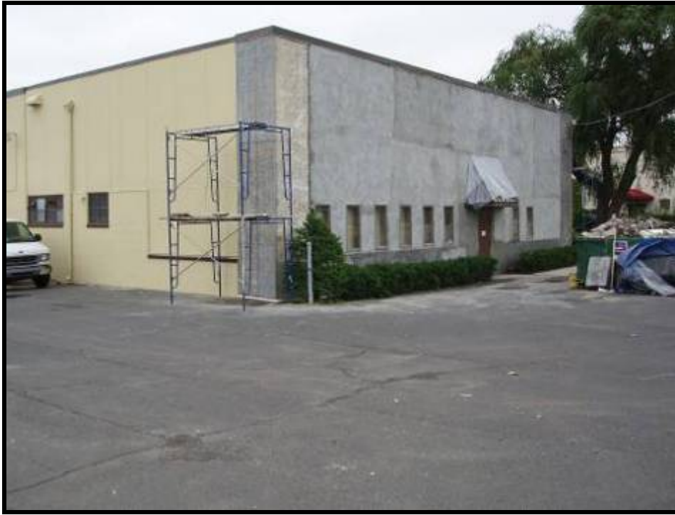
1. Looking at the front of 325 Washington Avenue (10/06/05)
