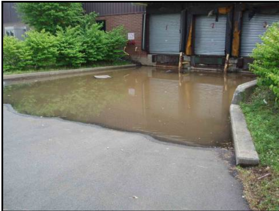
2. Flooding condition at loading docks on Madison Circle Drive (6/10/05)
