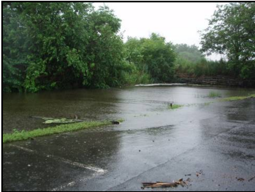
8. Flooding condition at 350 Gotham Parkway upstream of Peach Island Tide Gate (7/08/05)
