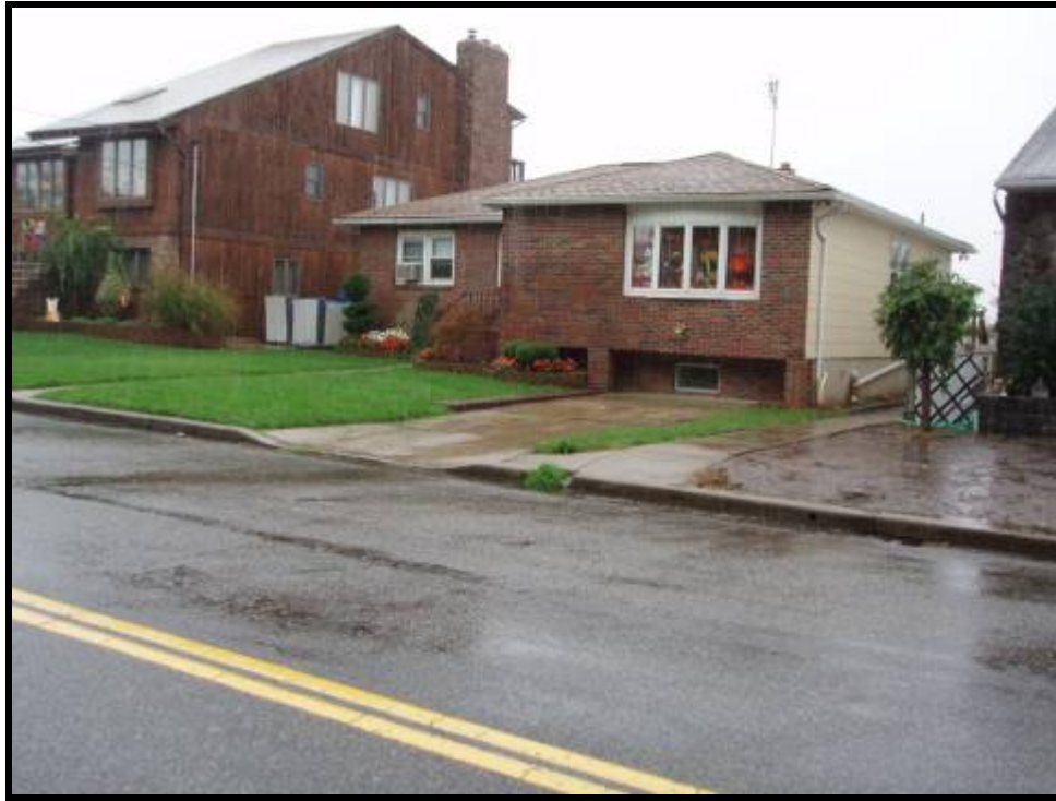
1. Front view of the property at 15 Mill Ridge Road (10/14/05)
