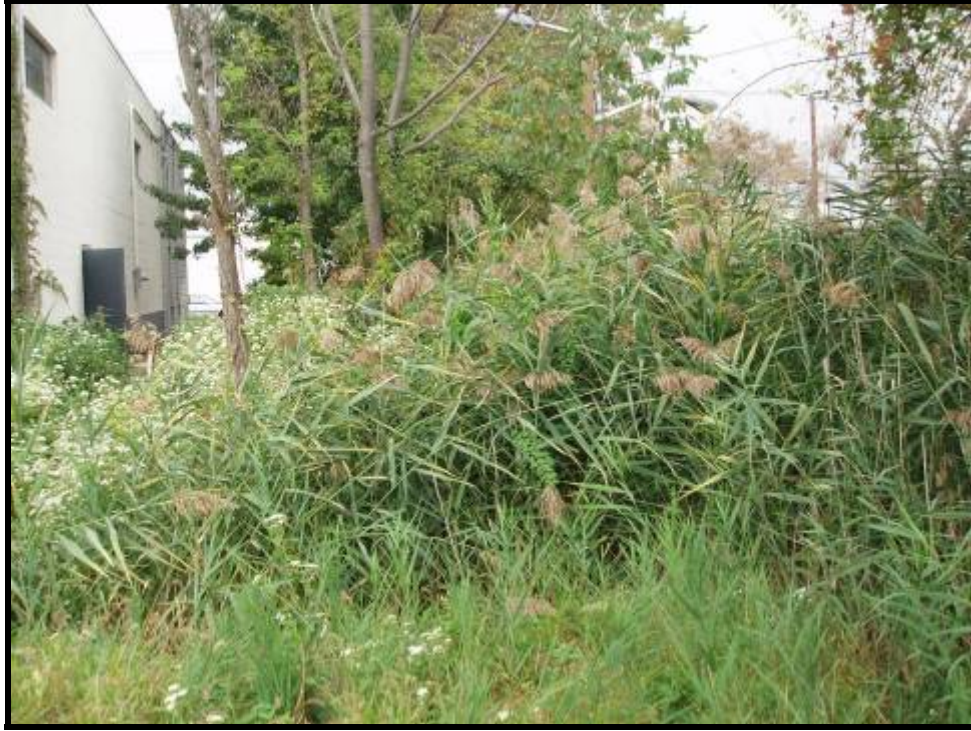
7. Drainage ditch at the rear of 654 Gotham Parkway (10/06/05)
