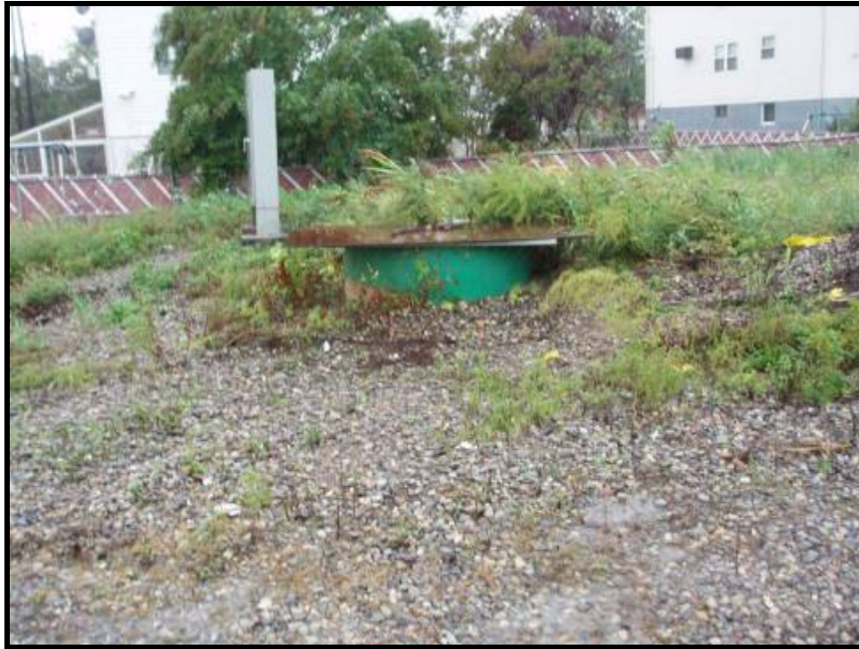
4. View of stormwater pump system located in the lot behind 64 Maiden Lane (10/12/05)
