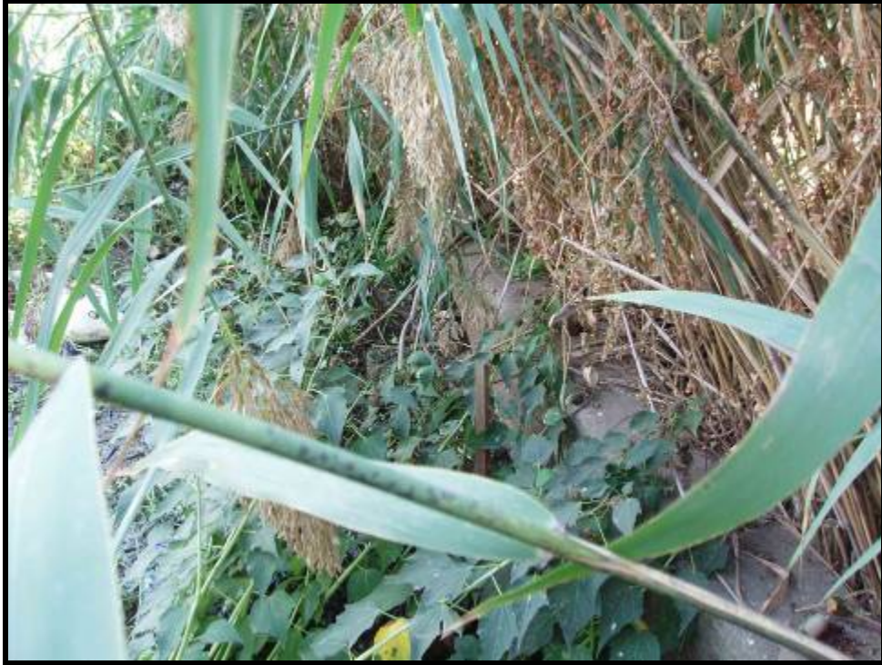
7. Headwall located underneath railroad, to pump station (10/06/05)
