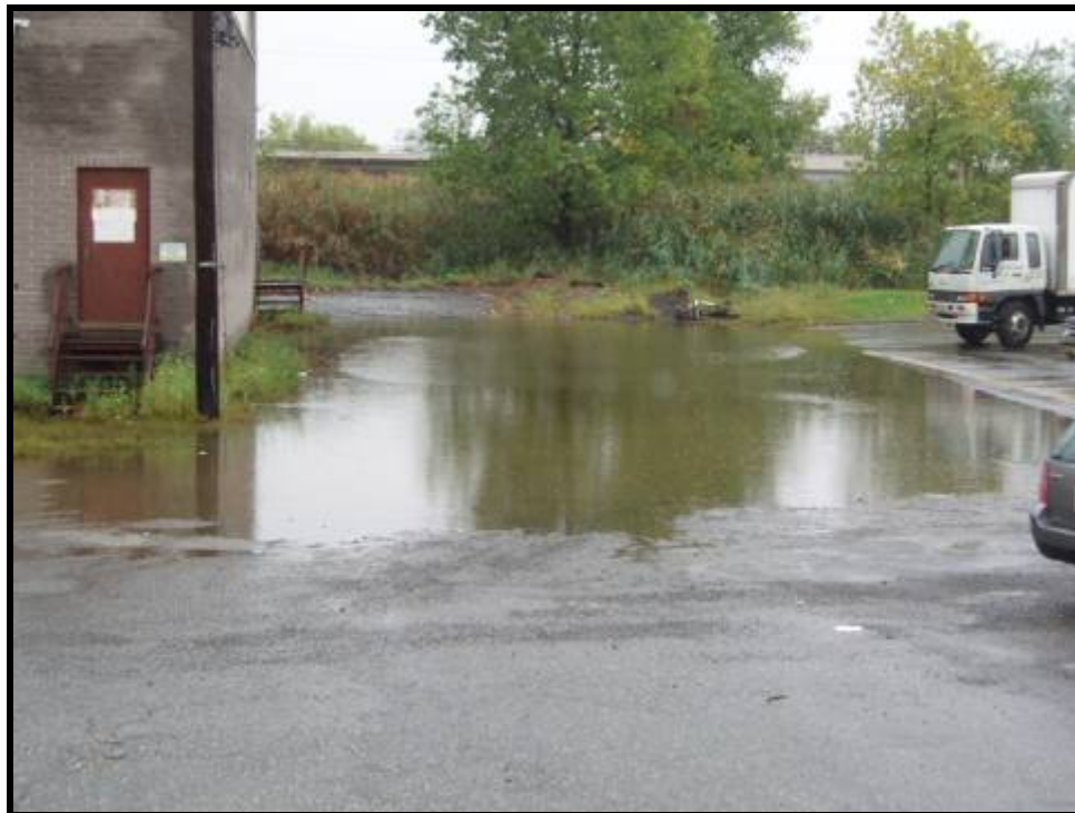
4. Flooding condition at 462 Barell Avenue (10/14/05)
