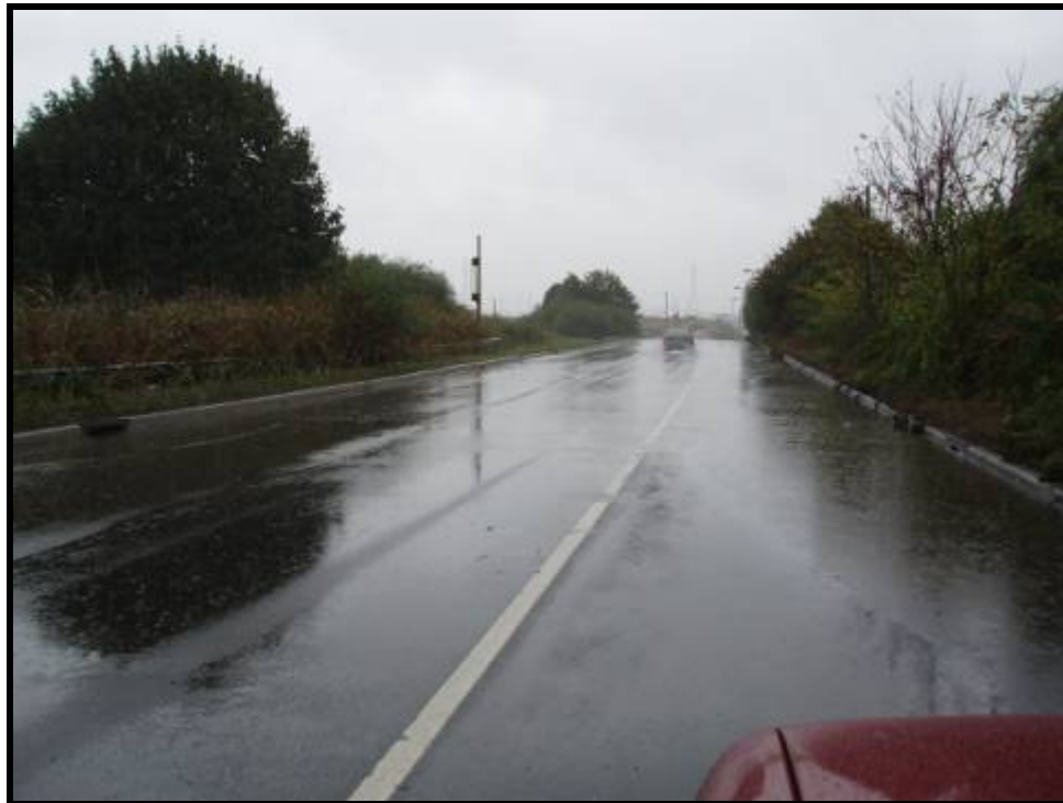
4. Ponding conditions on the shoulder of Belleville Turnpike (10/14/05)
