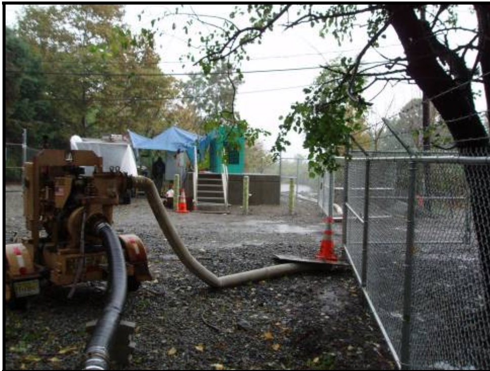
2. View of bypass pump system and new DePeyster Pump Station (10/11/05)
