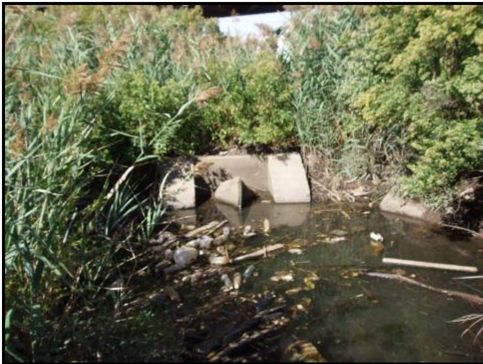
6. Second outfall with one-way valve system located alongside Fish House Road near CSX Rail Bridge (10/06/05)
