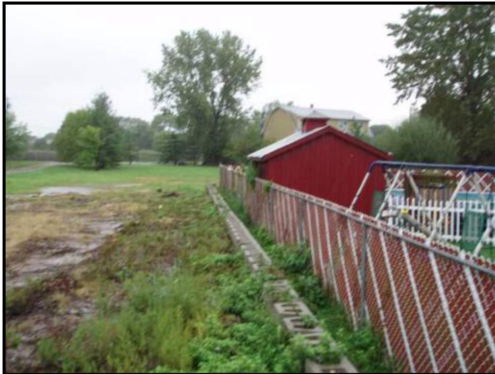
2. View of the retaining wall behind 64 Maiden Lane (10/12/05)
