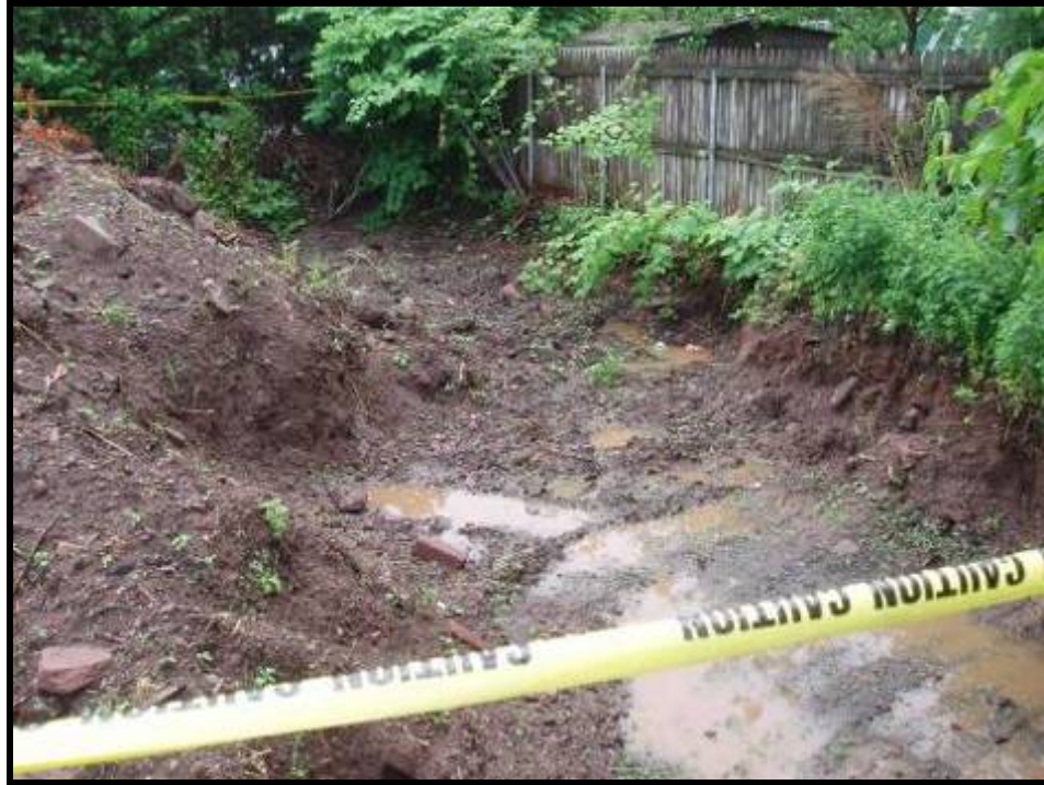
1. Infiltration basin located at 1600 Paterson Plank Road behind 1089 Farm Road (right) (6/10/05)
