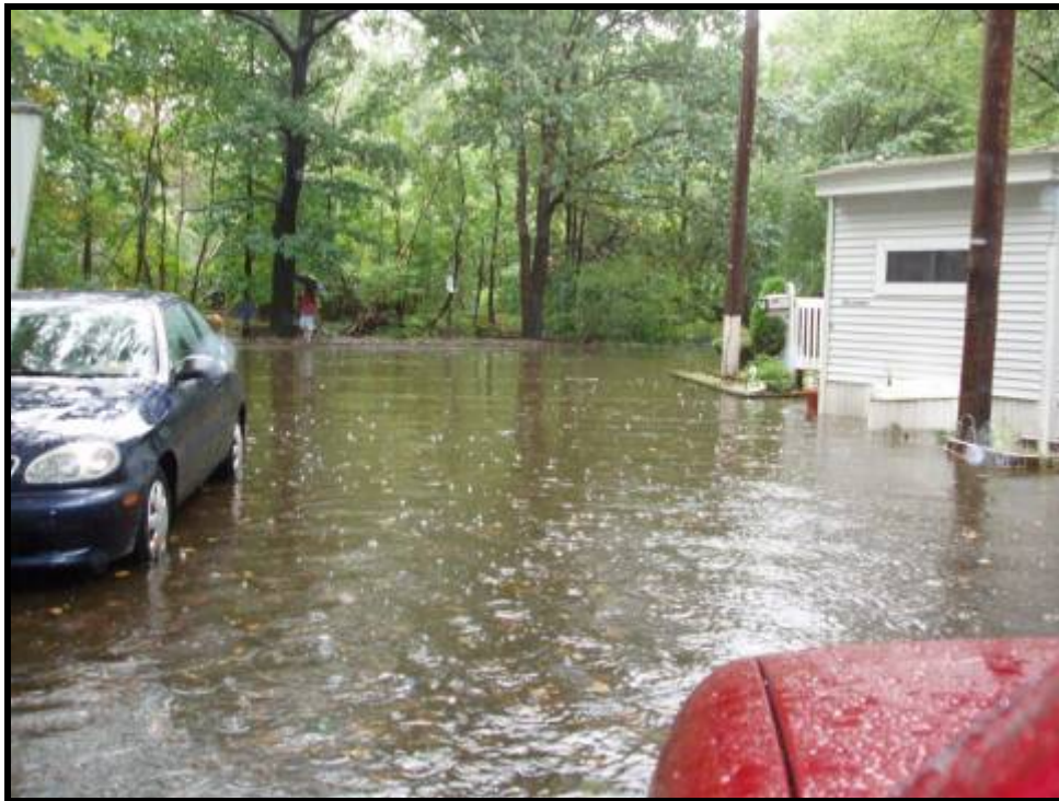
2. Flooding condition at Southeast of the mobile home area (10/14/05)
