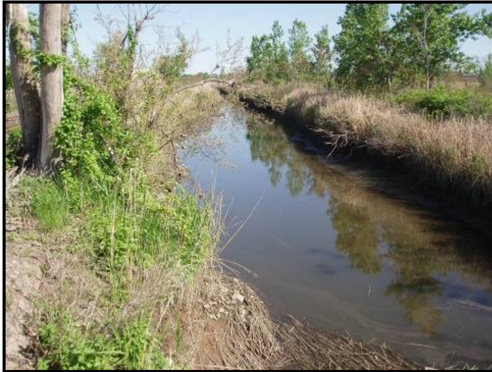
4. Drainage channel upstream of the Rutherford Tide Gates (5/17/05)
