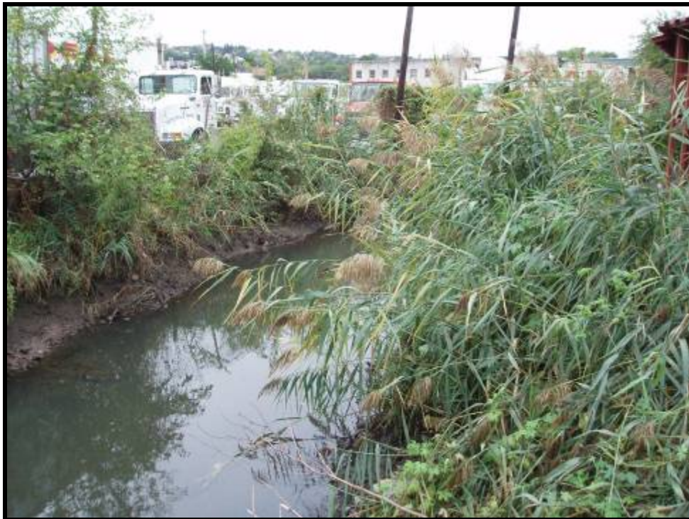
4. Looking upstream of Bellman's Creek at Fairview Avenue (10/06/05)
