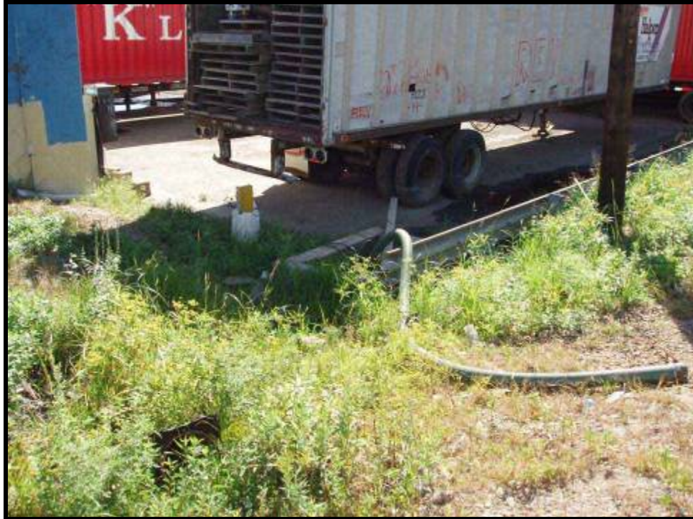
1. Make-shift pump system at 996 Belleville Turnpike (10/06/05)
