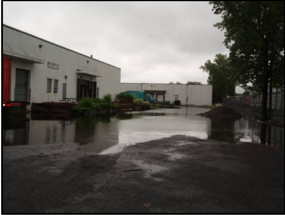
7. Flooding conditions at 745 Gotham Parkway in rear of the property (7/08/05)
