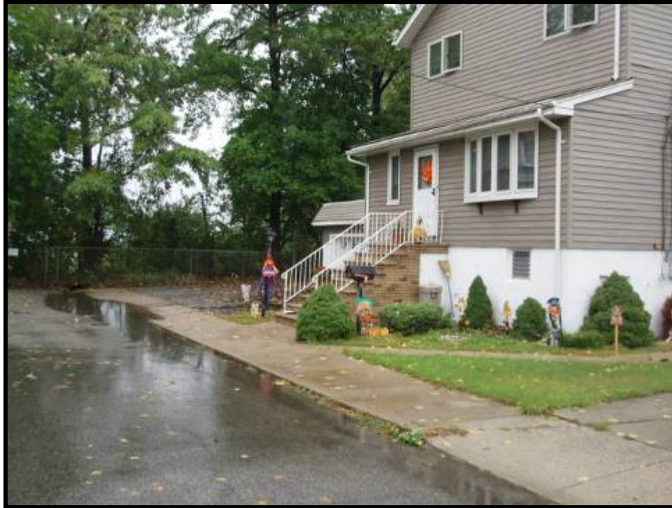
3. Front view of property at 37 Hartwick Street (10/14/05)
