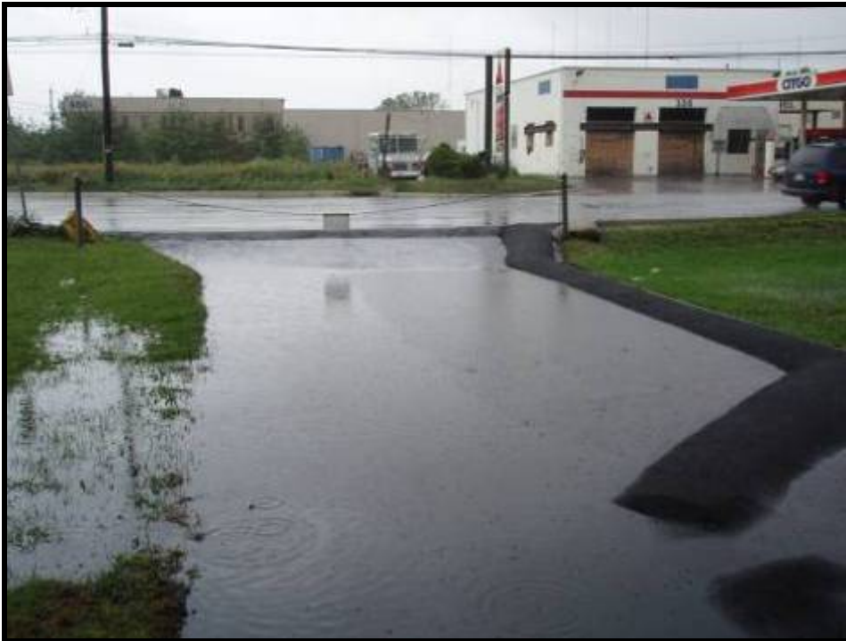
2. Looking at the raised berm and ponding of the driveway located at the south end of property (10/12/05)
