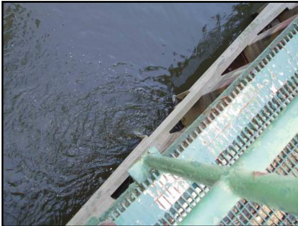
2. Boils observed upstream of West Riser Tide Gate during a tide change (10/06/05)
