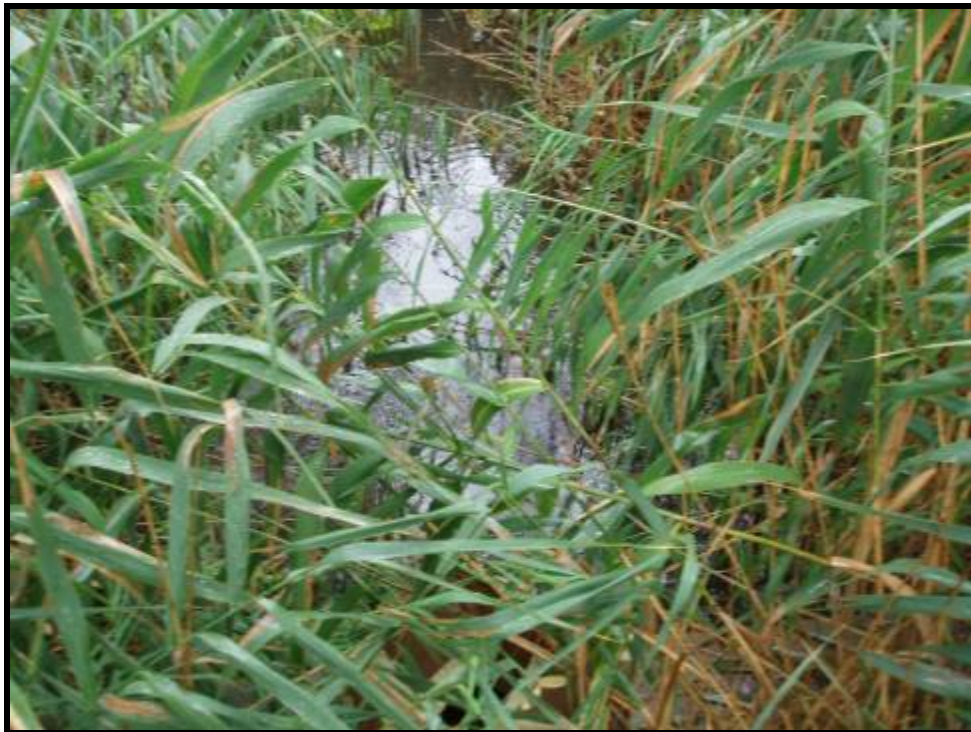
6. Looking downstream at the Michelle Avenue culvert (10/06/05)
