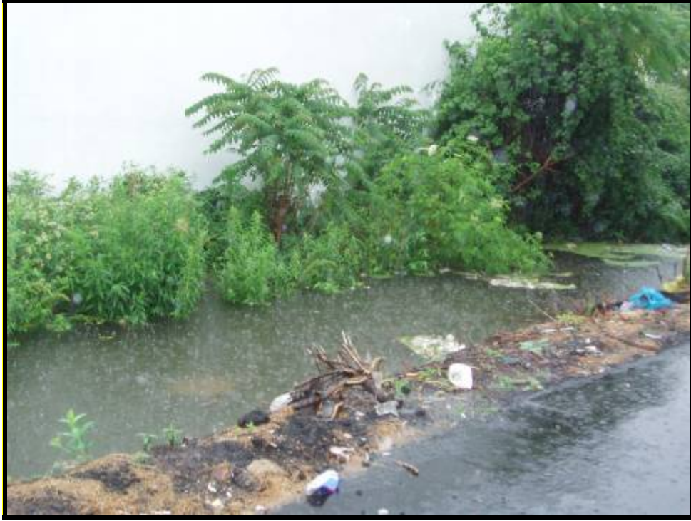
5. Drainage ditch behind 110 Asia Place (6/10/05)
