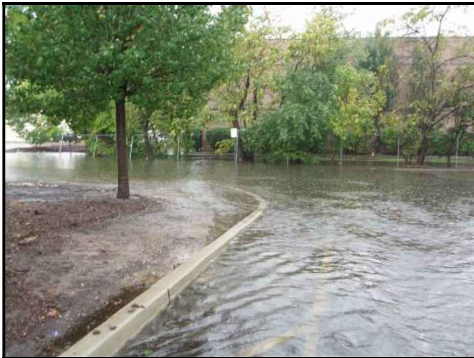
4. View of flooding in the parking lot at 1 Carol Place (10/12/05)
