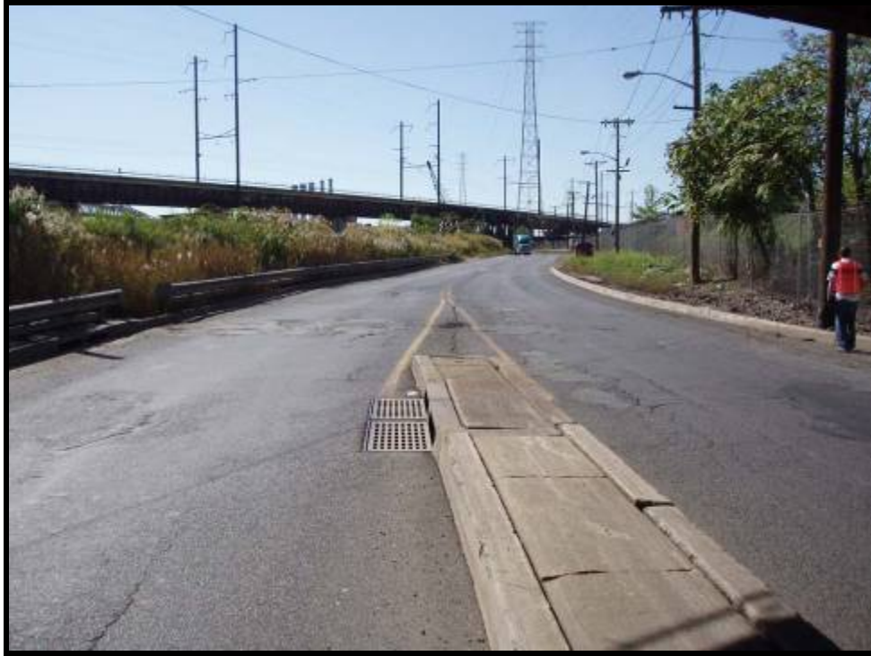
3. Looking West Along Fish House Road underneath the PATH bridge (10/06/05)
