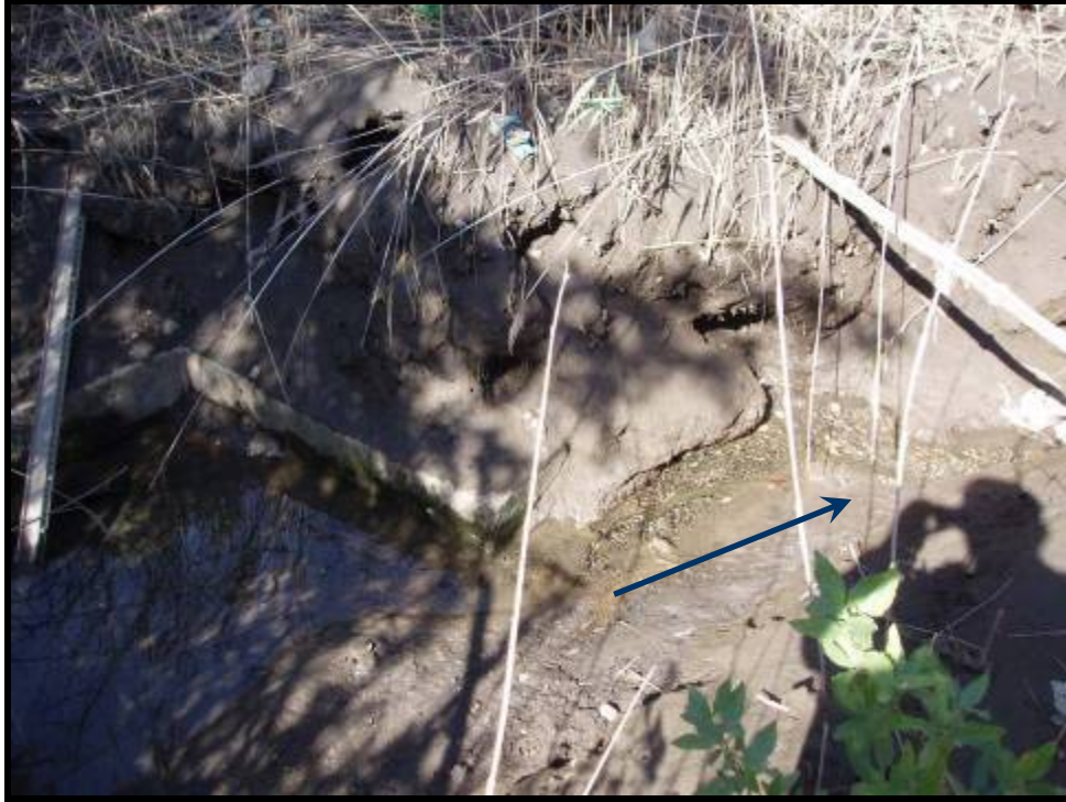
5. Drainage ditch serving system in Photo 4 (10/06/05)
