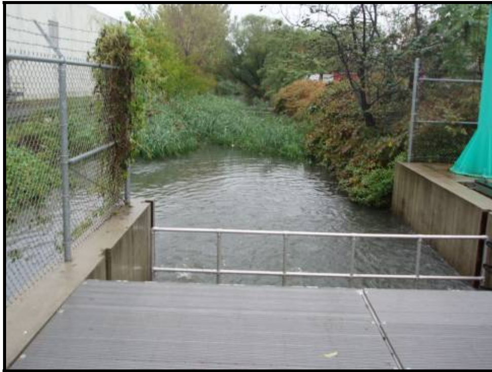
1. Looking downstream of Bellman's Creek at 91 st Street (10/14/05)
