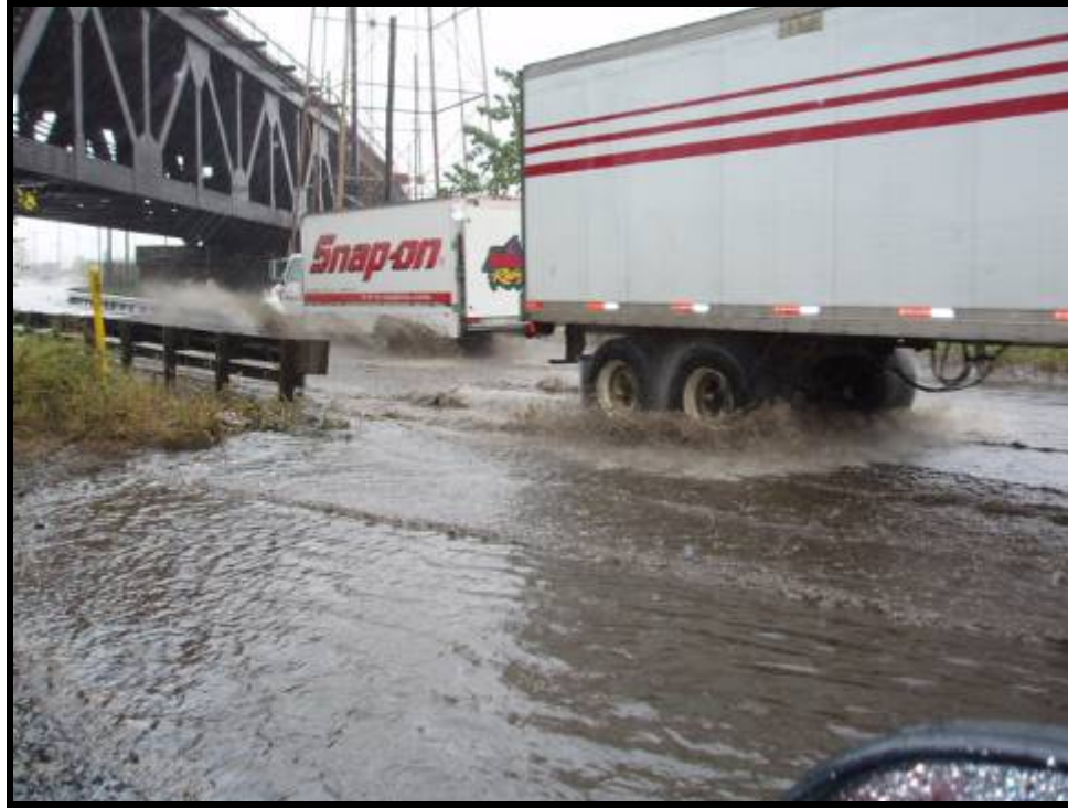
1. Looking Southwest along Fish House Road near the CSX rail bridge (10/14/05)
