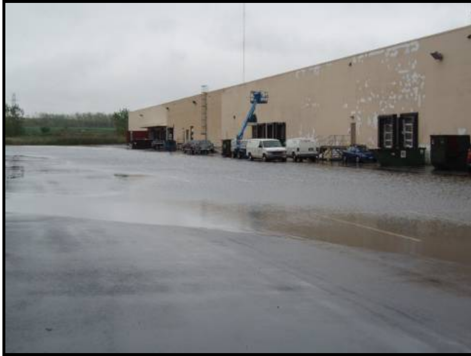
1. Looking southeast towards ditch at rear of property (10/14/05)
