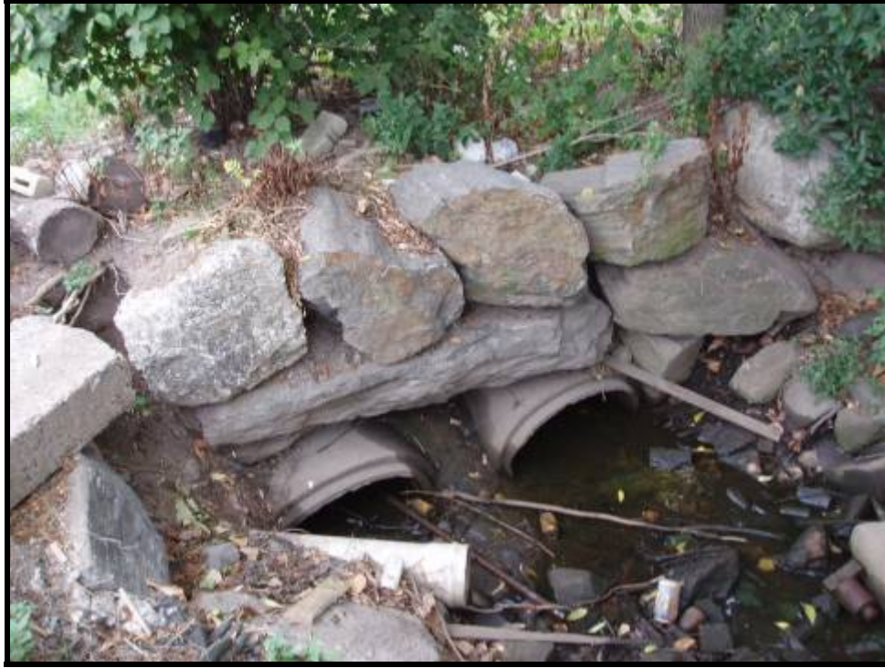
5. Elliptical culvert clogged with debris at the rear of 545 Dell Road (10/06/05)
