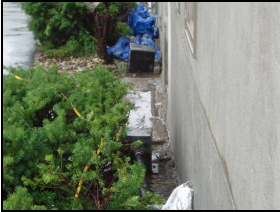
3. Two pump systems located in front of the building of 325 Washington Avenue (10/06/05)
