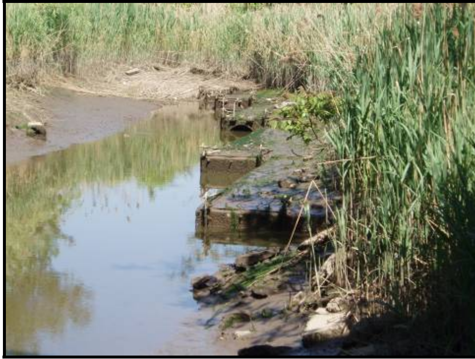
1. Looking Northwest at Rutherford Tide Gates outfalls (5/17/05)
