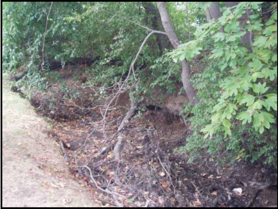
1. Drainage ditch at end of Carol Place (10/06/05)
