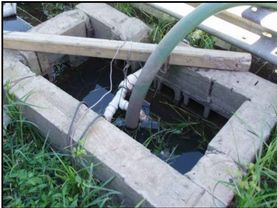
2. Sump pit for make-shift pump system at 996 Belleville Turnpike (10/06/05)
